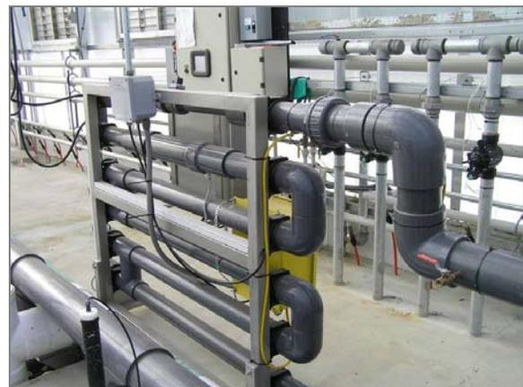
**Figure 9.3.** Installation of a copper ionization system in a commercial greenhouse operation.
