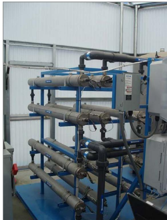
**Figure 11.3.** This ultraviolet light unit treats 100 gallons of water per minute and is equipped with high intensity bulbs (240 watts). Cost varies according to the water quality and the pretreatment that is required. Operating costs depend on the price of power. This unit requires 7.5 kilowatts to run.
