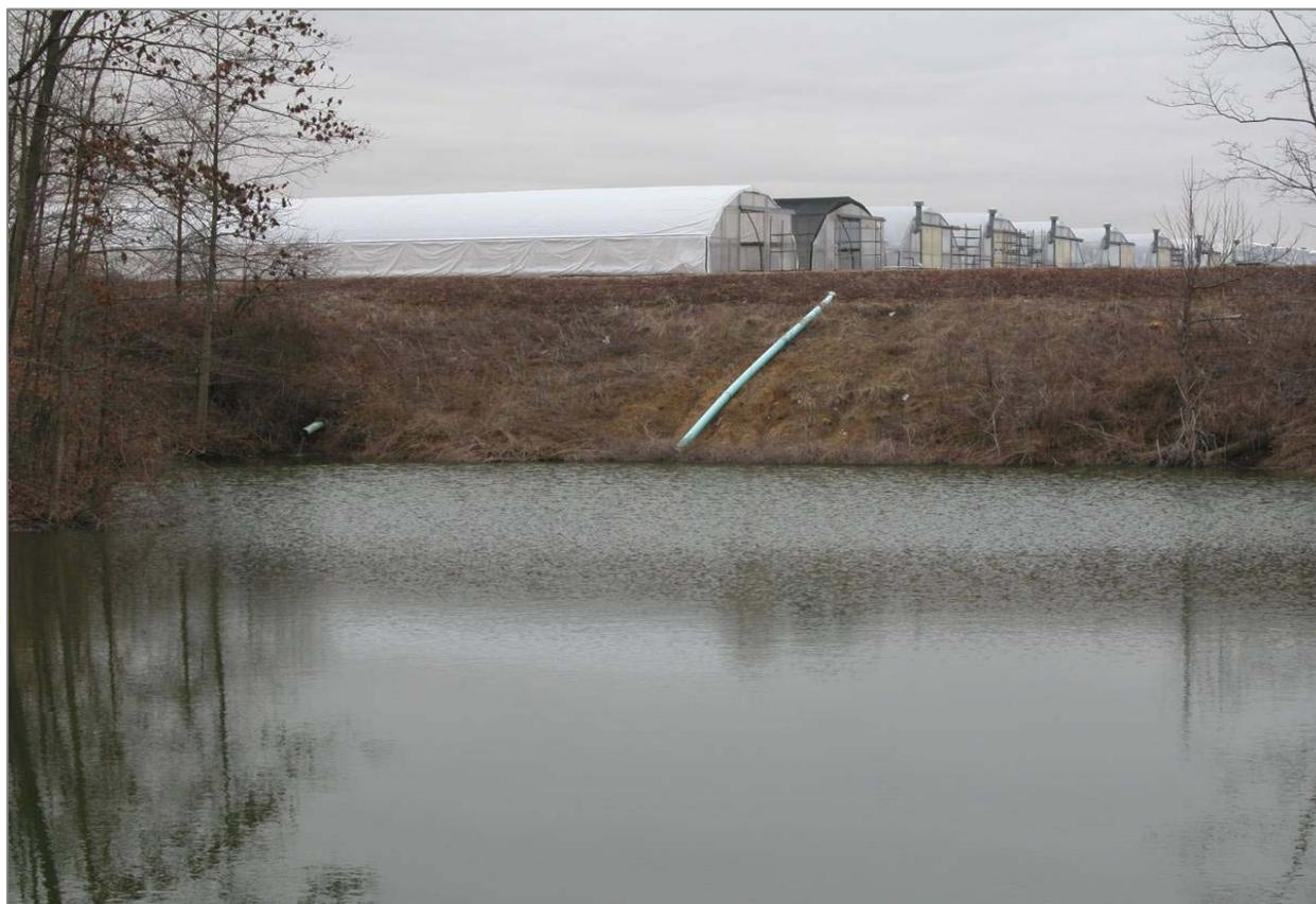
**Figure 3.1. Containment ponds are increasingly being required by water management authorities to capture runoff and store irrigation water.**
