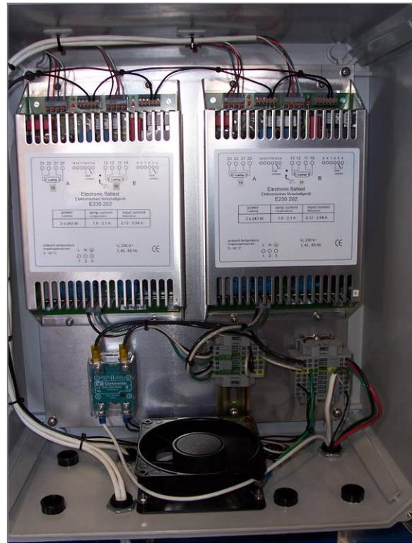
Figure 11.1. Two electrical ballasts, each drives two ultraviolet light bulbs.
