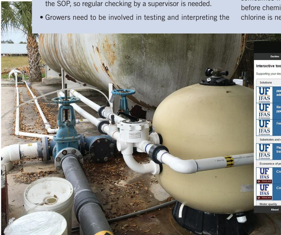
**Figure 2.** Pond water was passed through a sand filter (bottom right), dosed with liquid bleach (bottom left), and held into a tank (background).
